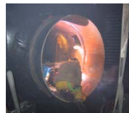
Clearview Water Line being constructed.
