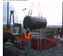
Clearview Water Line being installed.
