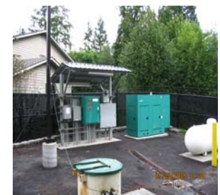
2004 lift station improvements.
