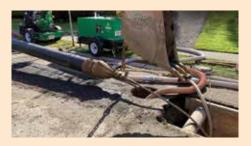
This technique starts with a conical metal "battering ram" head attached to the leading end of the pipe, and then connected with a steel cable through the existing pipe to a hydraulic jack on the other end.
