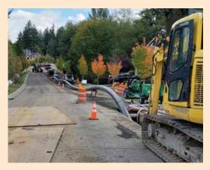
Three flat sections of 8-inch sewer pipe flowing into the existing Sector 7 Lift Station needed to be upsized to 12-inch for greater capacity. Two of the shallower sections were dug up and replaced using traditional open trench construction methods, but the deeper middle section was replaced using a new pipe bursting technique.
